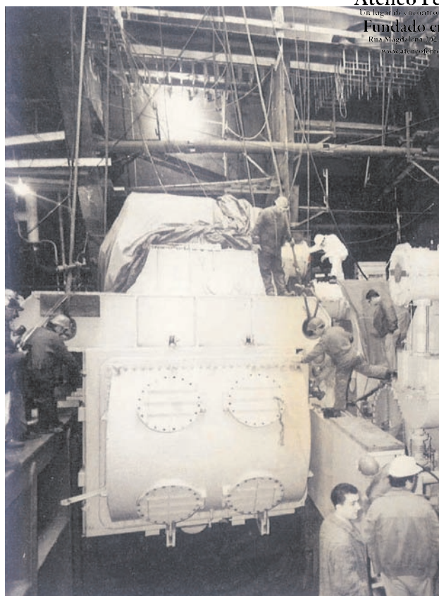
▲ Ensamblando as turbinas, ASTANO (1972).
